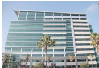
The city has issued two stop work orders on construction of the top two floors of a 12-story office building in Kearny Mesa.
