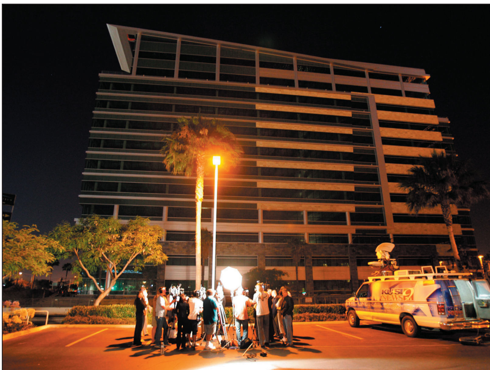
At last night's news conference outside the Sunroad office building under construction in Kearny Mesa, an attorney for Sunroad Enterprises said the company will lower the tower to comply with federal aviation height limits. Sean M. Haffey / Union-Tribune photos
